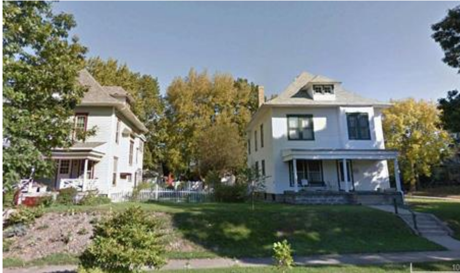
3338 Brookside Parkway, Indianapolis. 1943-1950
